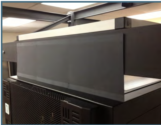
Fill Gaps Above Racks
