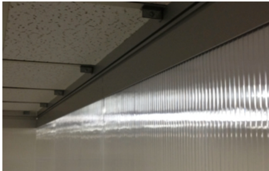
Support Channel attached with P-Clips
